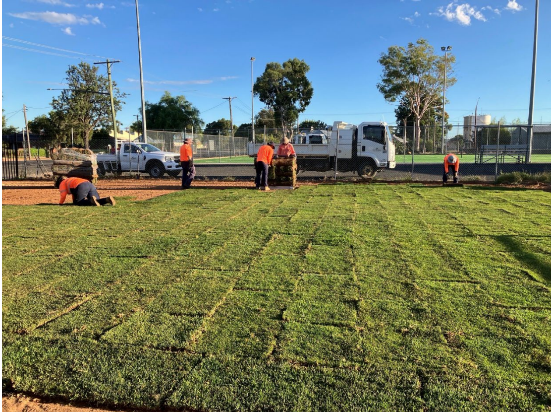
Figure 6: New Turf installed at Cale Over
