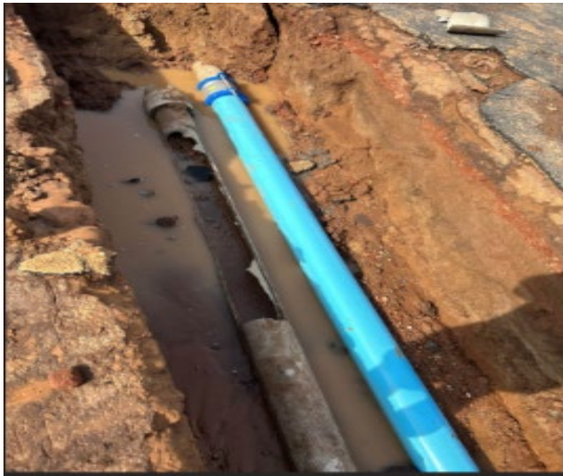
Figure 1: Replacement water main in Temoin Street
