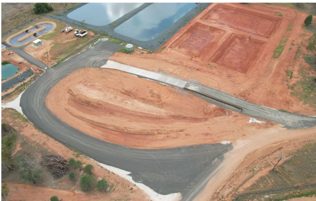
Figure 9: Aerial view of Trangie Truck Wash
