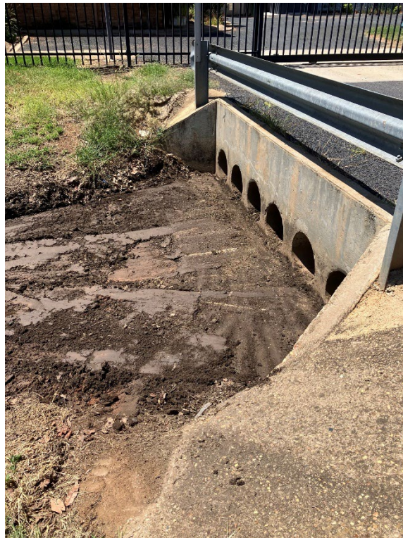
Figure 7: Stormwater drain cleaning occurred across Narromine in February
