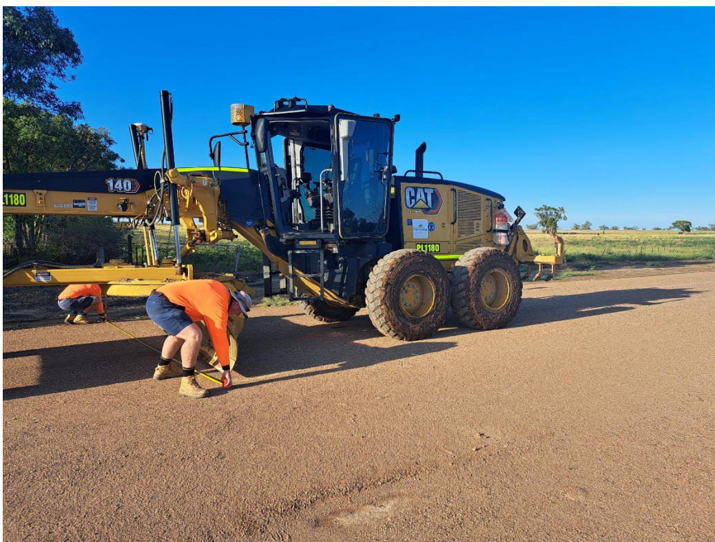
Figure 8: One of Council's grader teams inspecting the road width
